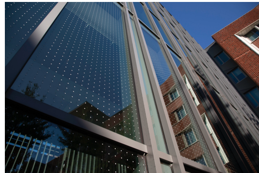
Bird-friendly glass at The Audubon Discovery Center in Philadelphia, Pennsylvania. Photo credit: Luke Franke.
