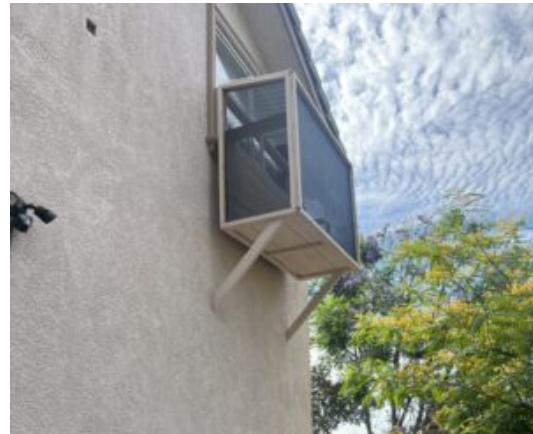
A window-box catio which is secure for both birds and cats with a thin-meshed pet screening that does not allow critters or birds to enter.
