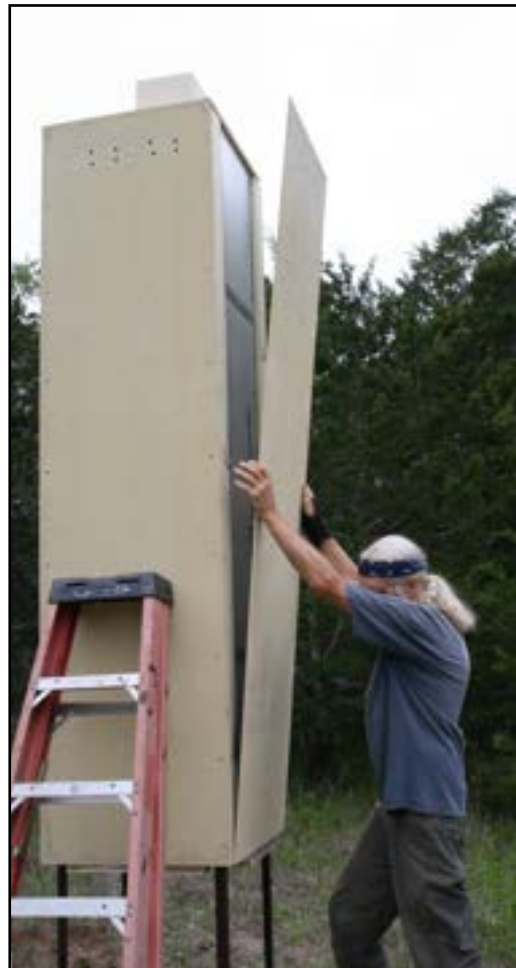
Figure 18 - installing Hardie panels
