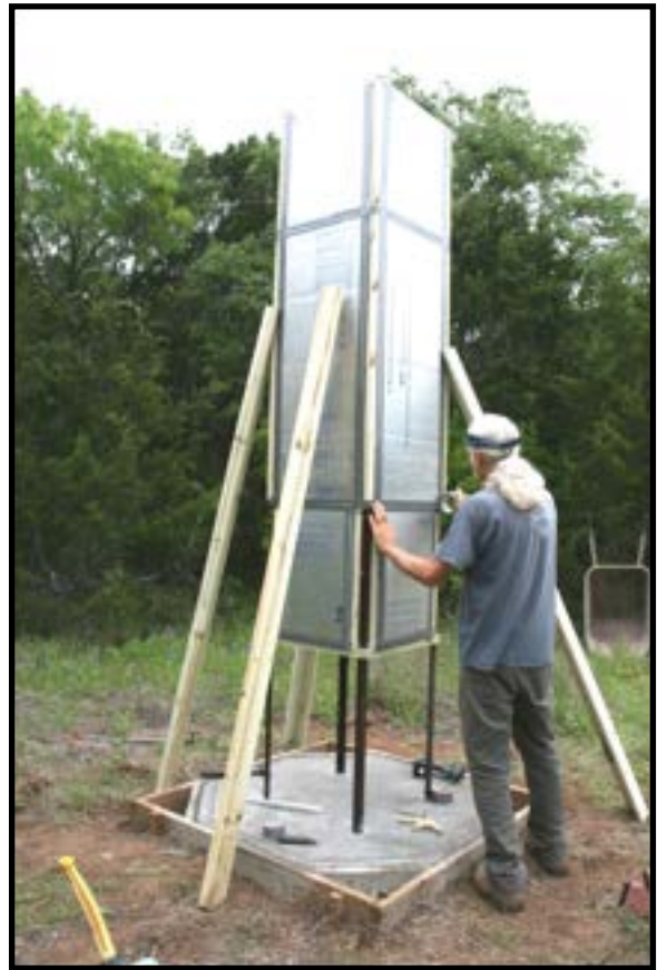
Figure 14 - installing the Insulation Panels
