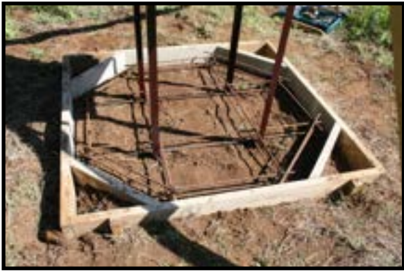
Figure 10 - foundation form, tower legs and rebar ready for concrete
