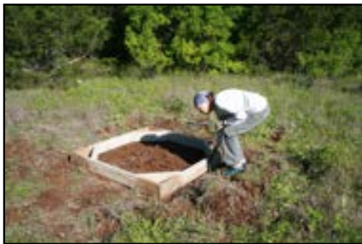
Placing the Form Box
