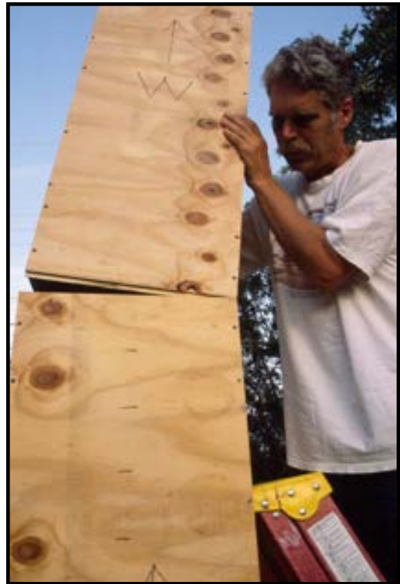
Figure 12 - installing the top section of the Nesting Chamber
