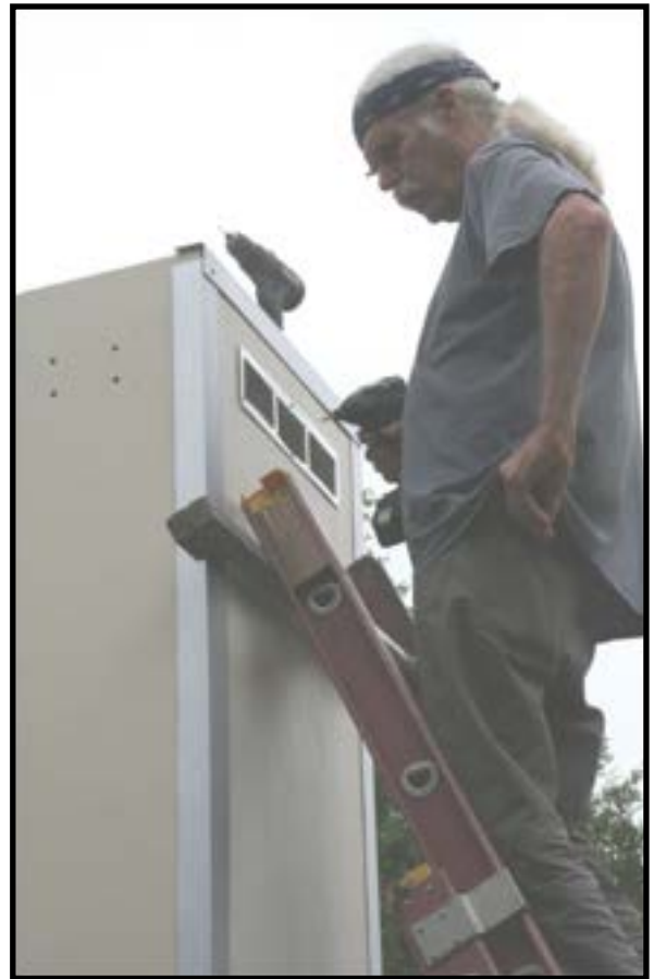
Figure 19 - installing Soffit Vents
