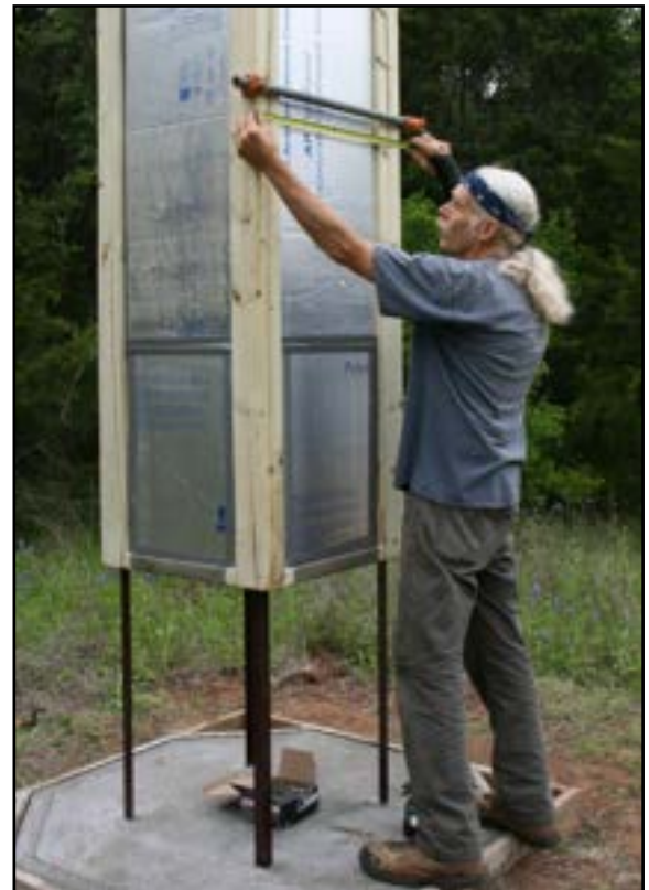
Figure 15 - installing the Wide Outside Corners
