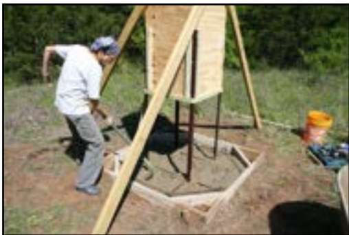
Spreading and tamping the concrete
