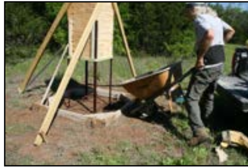
Pouring the concrete
