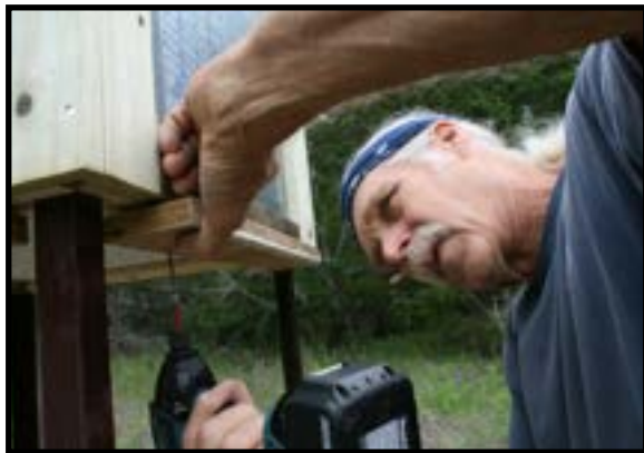
Figure 17 - installing Hardie support shelves
