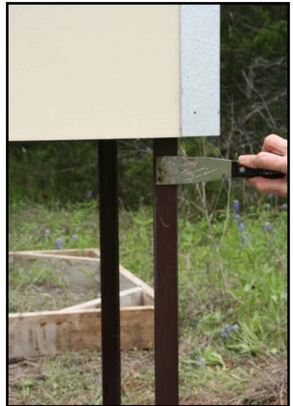
Figure 20 - installing Tanglefoot insect barrier
