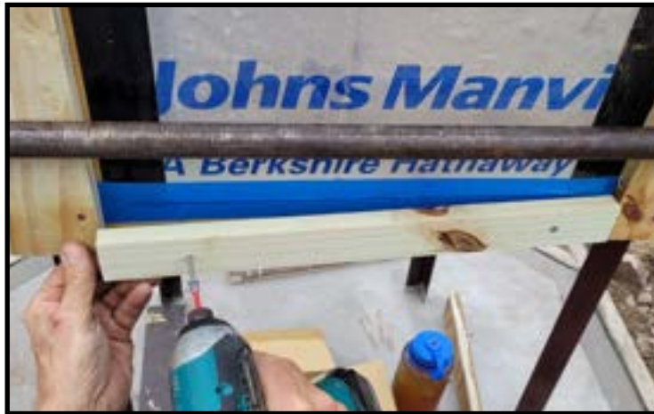
Figure 16 - installing the 16 7/8" Outside Horizontal Bottom Cleats
