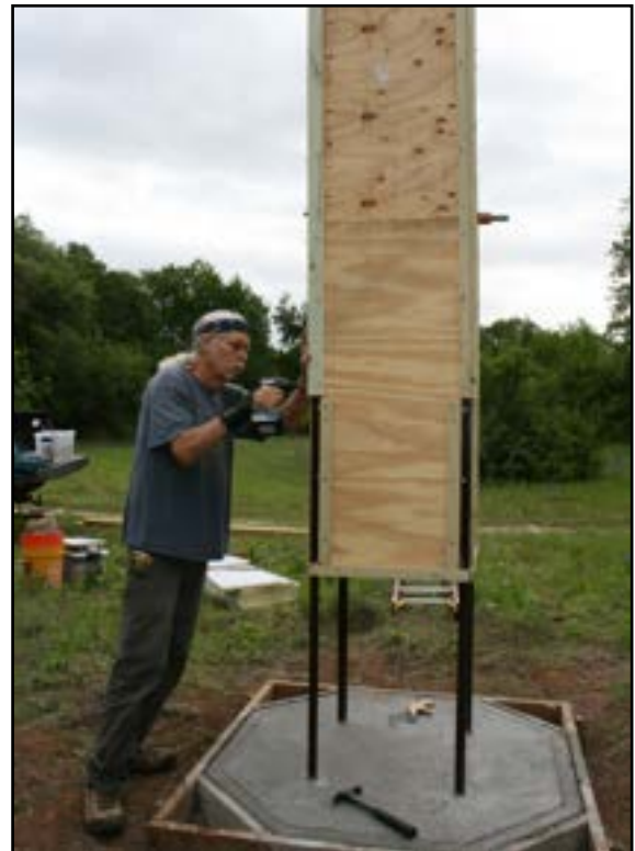
Figure 13 - installing the Narrow Outside Corners
