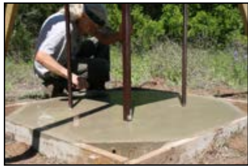
Leveling the top of the foundation
