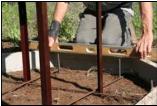
Checking for level and rebar pin height
