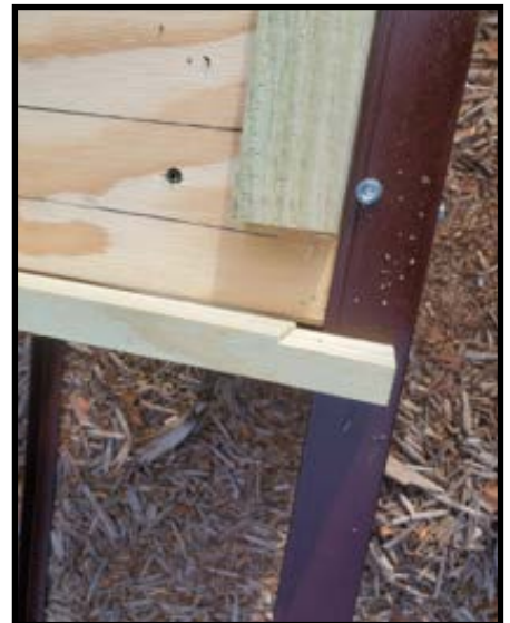
Figure 5 - bottom cleat showing notch
